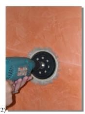
WORKING TEMPERATURE OF BOTH THE ENVIRONMENT AND THE SURFACE: 7°C minimum and 32°C maximum
